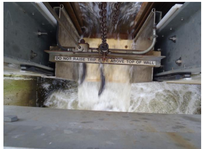
Two shad slide down the chute at the Greenville Dam Fishlift after being lifted with ~20 of their closest friends. After dropping a foot into the exit flume, the fish will swim past a viewing window to be counted.
